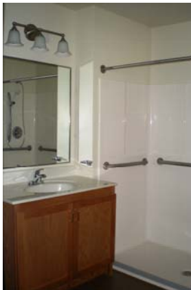
Above: Partial view of bathroom in a consumer apartment
